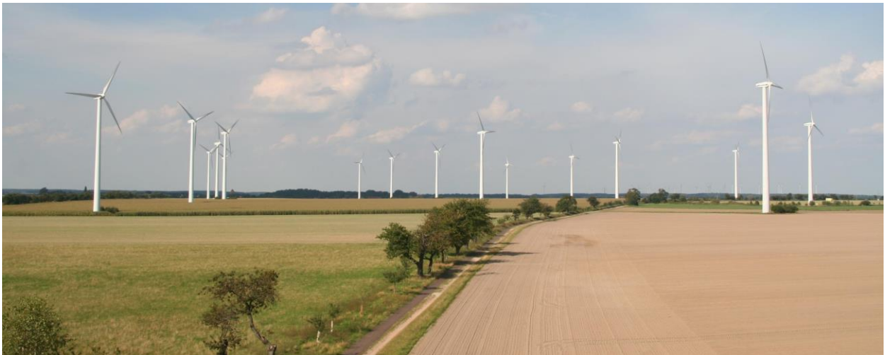
Abb. 8: Windpark Deetz, MILAN-Bild, Seehausen
